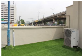
MTN PLAZA - WALKWAY PROJECT.
